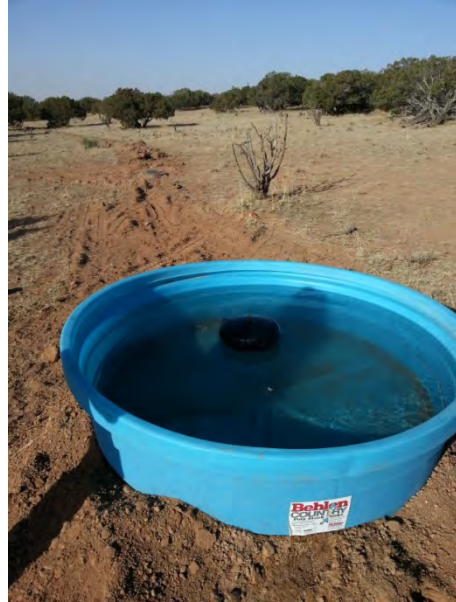
End of livestock pipeline-drinking tub
